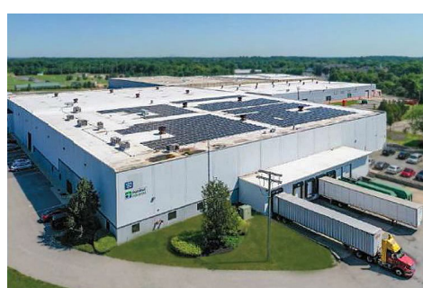
INDUSTRIAL High Hill Rd Swedesboro, NJ Acquisition of a 107K SF single tenant industrial warehouse located in Gloucester County, NJ.
